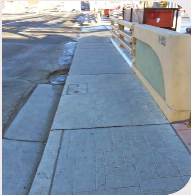
Figure 2.6 - Narrow sidewalk at the bridge crossing I-80
