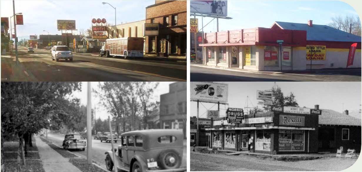
Figure 4.3 - Virginia Street before, during and after widening (pictures courtesy of Barry O'Sullivan)
