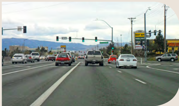
Figure 5.2 - Virginia Street and South McCarran Boulevard intersection
